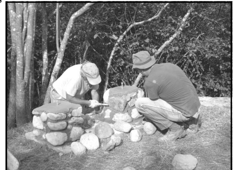
Master mason John Viselli and students built benches and a waterfall for the memorial park.
