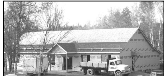
Commons under construction—November 2006
